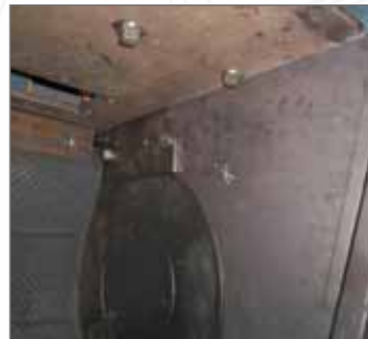
Tumble Blast Rebuild
